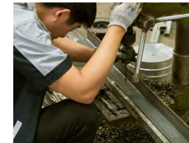
3 Angle Steel Punching
